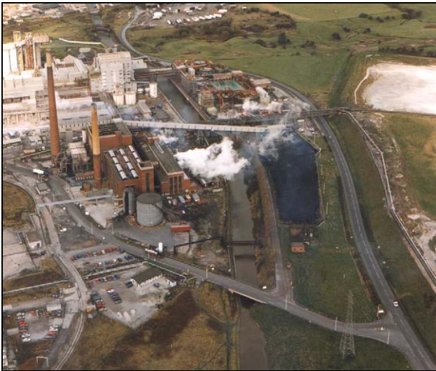
Figure 3.6: The Redundant Power Station Building, Looking North Across The Site
