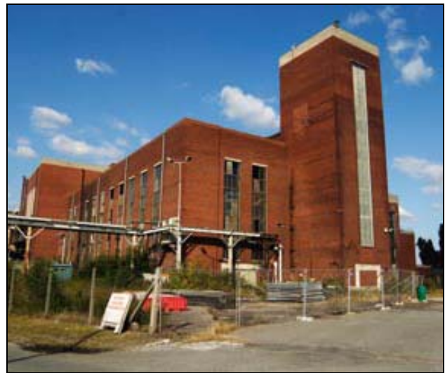
Figure 3.7: The Redundant Power Station Building, Southern Elevation
