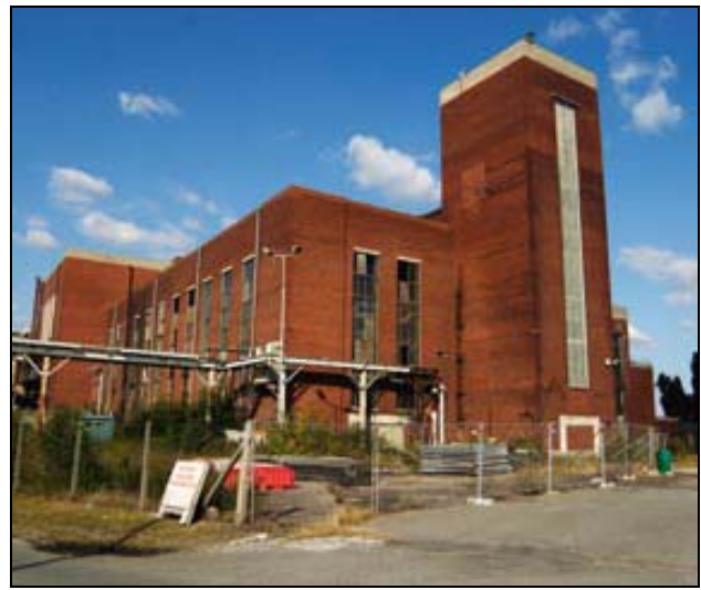
Figure 3.7: The Redundant Power Station Building, Southern Elevation
